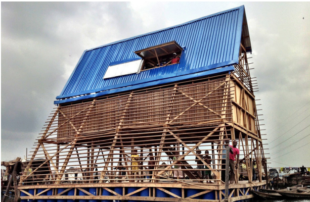
Figure 44: Makoko floating school timber structure.
