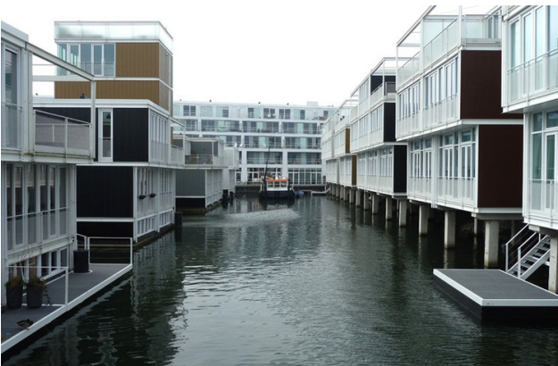
Figure 59: The picture shows houses constructed on pillars on the right and totally floating houses on the left.
