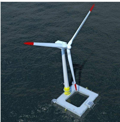
Figure 77: IDEOL floating structure
