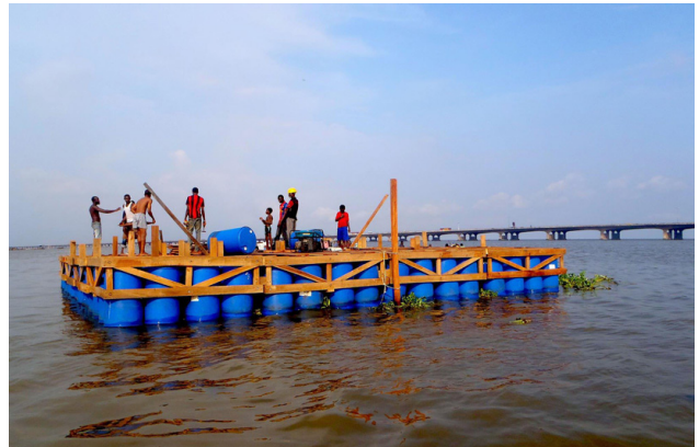
Figure 45: A floating foundation of plastic drums.
