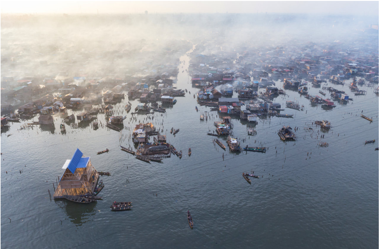
Figure 43: An aerial view of Makoko floating school within the context of the waterfront community in Lagos
