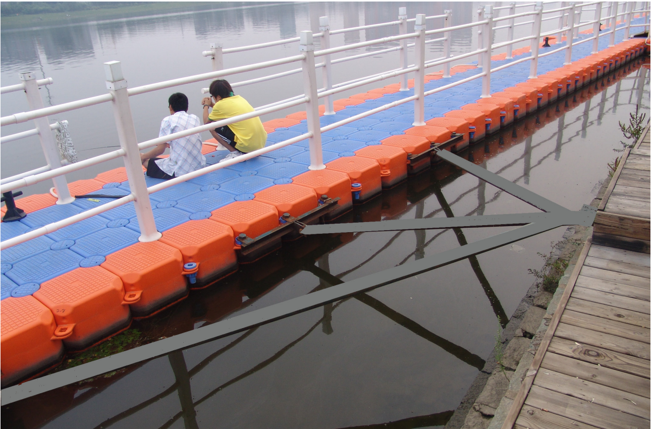
Figure 91: A picture showing a mooring system technique that can be used in the connecting floating units to nodes.
