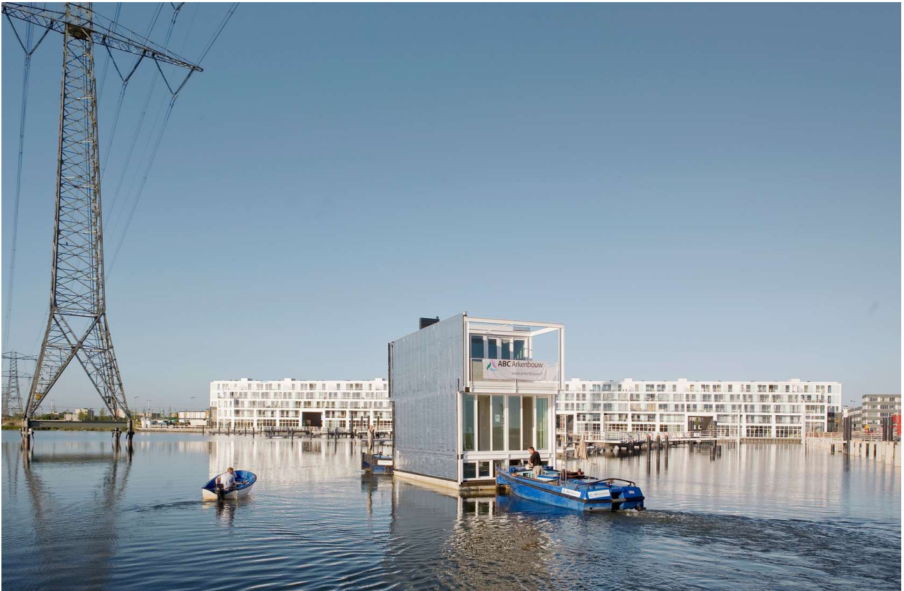
Figure 56: A floating house being towed into position. Houses are constructed in a shipyard and floated to site.
